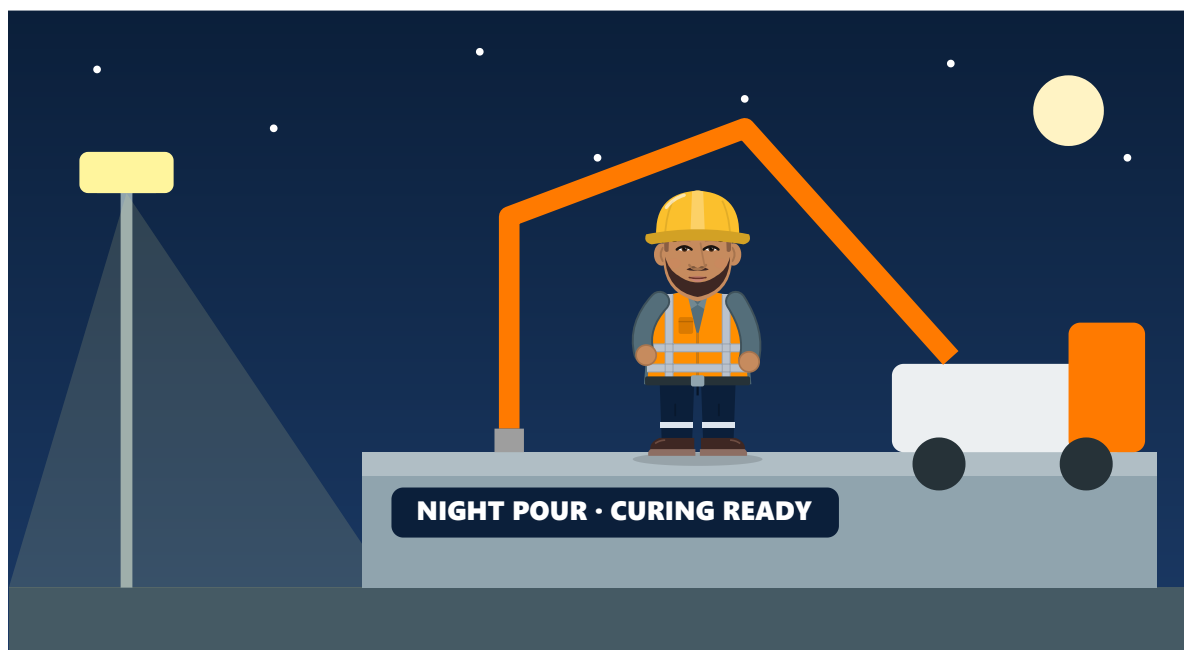
Night concrete pour with pump, lighting and curing hessian ready
